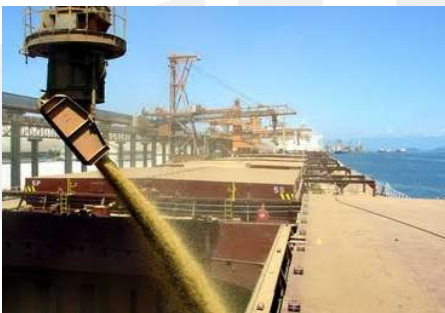
Paranaguá Bulk Terminal
